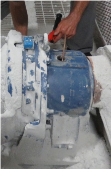
Figure 1: Oil sampling on in-line gearbox.
