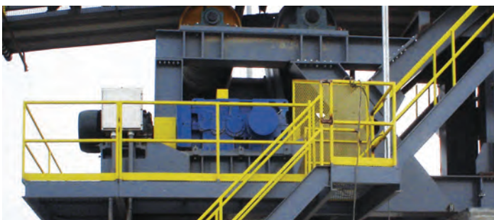
Paramax conveyor drive
