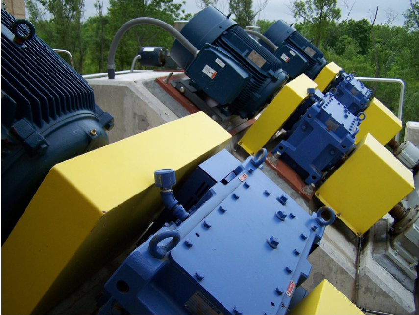
Figure 10: Screw pump applications require a 38° angle of inclination.
