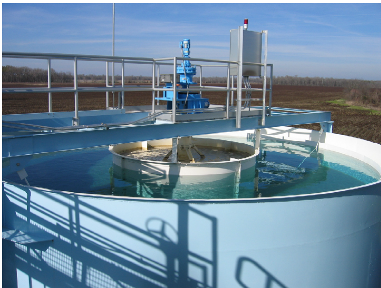
Figure 7: The same unit now installed at the center of a large clarifier tank
