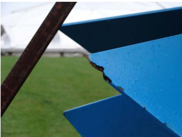
Figure 8. Example of Broken Impeller tip for Aerator 1
