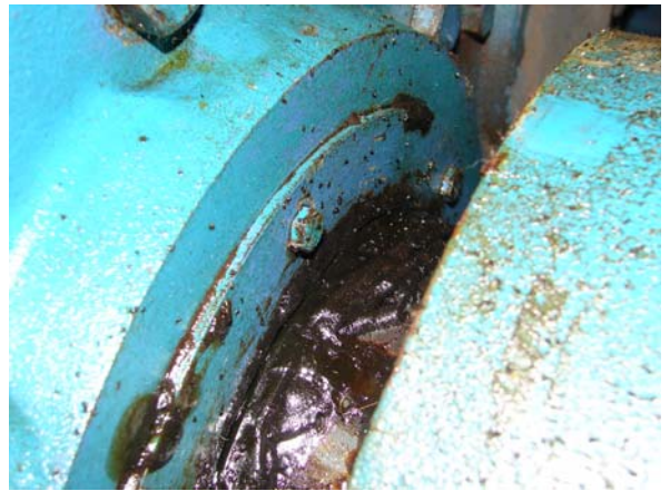
Figure 10. Low Speed Seal Area at Factory Inspection
